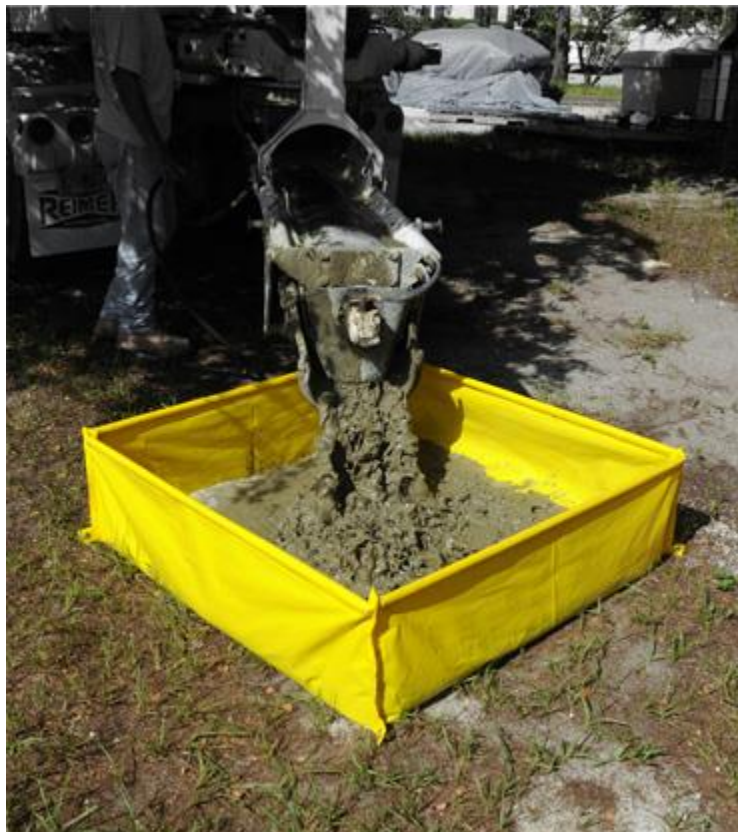
Figure 7 - Temporary Concrete wash-out area with impermeable liner
