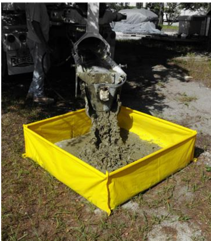
Figure 7 - Temporary Concrete wash-out area with impermeable liner
